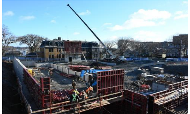
Foundations & Stairwell Construction
